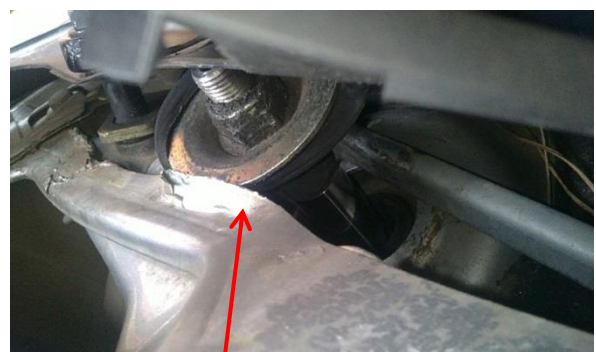
Low quality suspension bearing and insulator assembly
